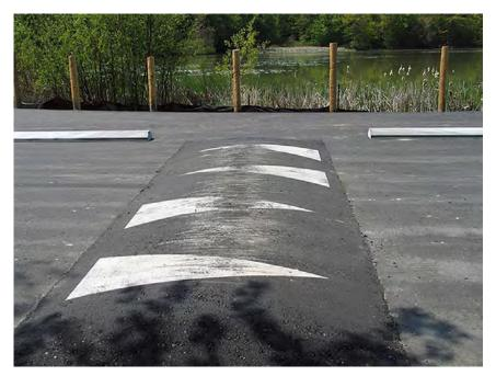
Asphalt speed humps can be installed along Peninsula Road to prevent speeding through the study area. Ideally, these would be placed near crosswalks or intersections to protect pedestrians. These would be a permanent fixture and lost if any upgrades were done to the Peninsula Road.
